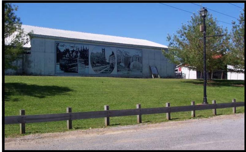
Above: Example of Short Term Recommended Improvement #3: replacing steel guard rails with wooden barriers. This example is from a village parking lot, Lyons, NY.
