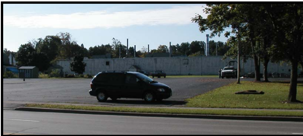
Above: Existing parking lot and Prestolite facility
