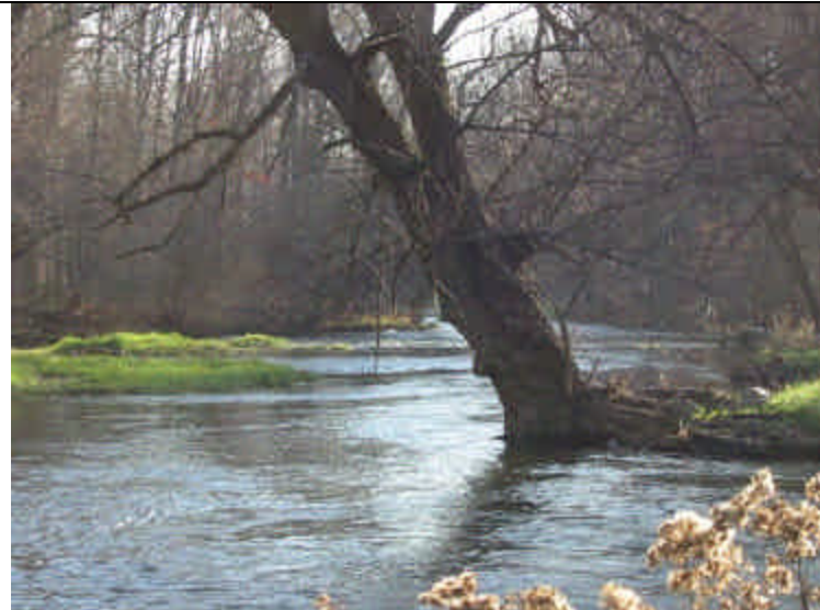
Single remaining black willow tree holds bank in place. Root system is completely exposed.
