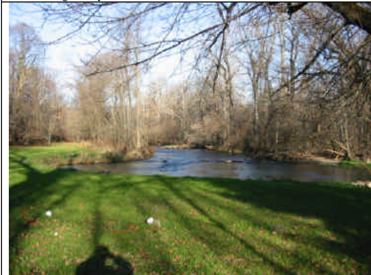
View of south bank of Oatka Creek, looking west (upstream) from leaning willow tree in photo above. Current has scoured a large indentation in the south bank.
