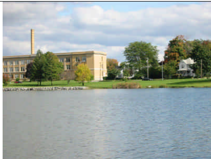
Photo 2. View of south bank of Oatka Creek, with Wolcott Street in the background. Note partial stone riprap along bank at photo left, and growth of riparian vegetation (bur-reed) at photo center.
