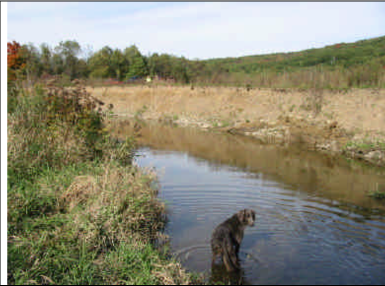
View of Oatka Creek exposed soil bank near Station 2+38, looking north.
