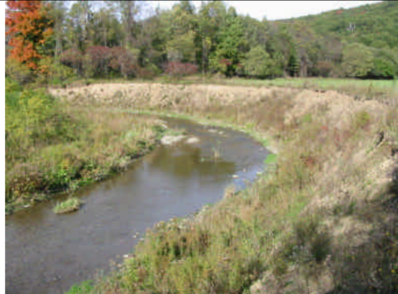
View of exposed soil bank at Station A0+800, looking northeast.
