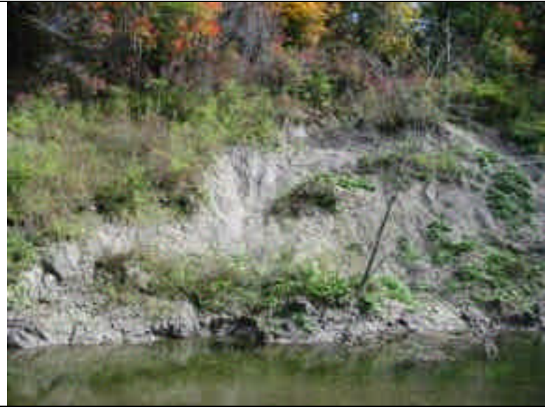
Detail of eroding bank in photo at left. Deep pool in stream channel undercuts clay bank, causing rotational slumping. Re-direction of channel flow away from this bank is needed to allow stabilization.
