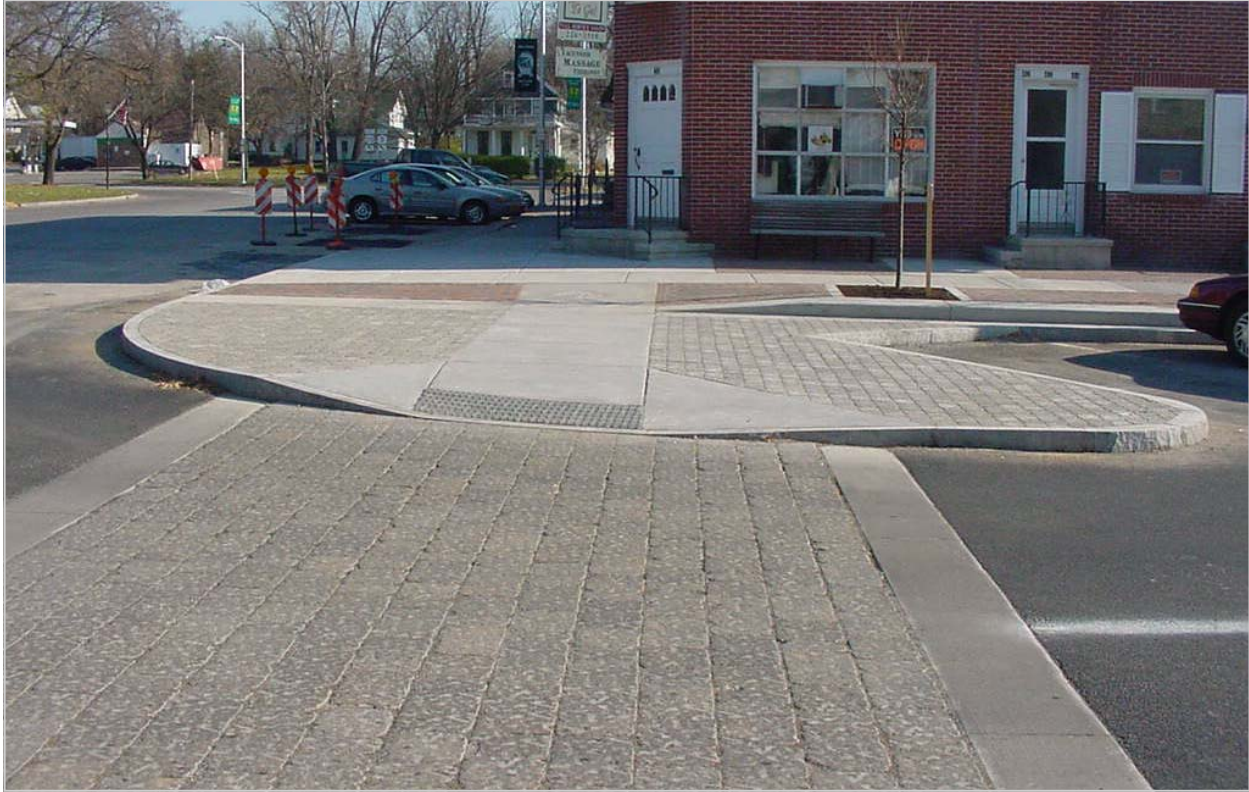
The combination of an enhanced crosswalk and curb extension installed on Main Street (NYS Rt. 20) in Avon, NY increases pedestrian comfort and safety and serves as a reminder to motorists to slow down. Source: NYSDOT Region 4
