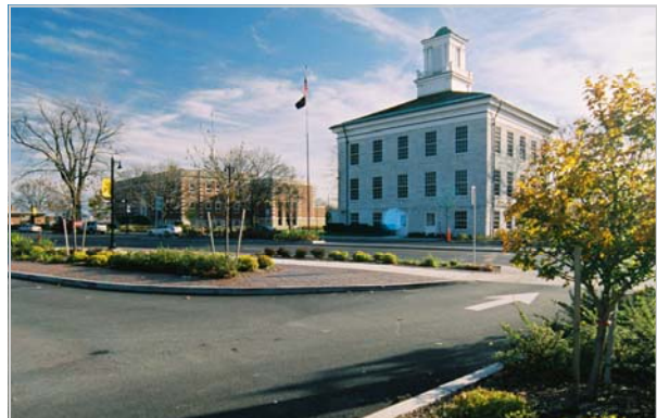
The multi-million dollar road construction project in Batavia, NY was completed in 2004 and has been recognized as a major success. This and other regional projects are featured in the report. Source: City of Batavia DPW
