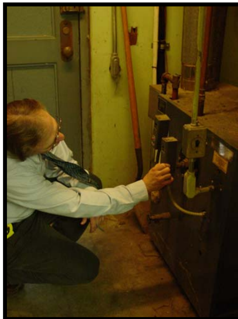
Wayne Balas, CJ Brown Energy, inspects the boiler at Victor Village Hall
