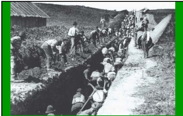
1874 – Construction begins on pipeline to deliver Hemlock Lake water 29 miles to Rochester
