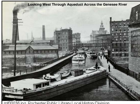
Looking West Through Aqueduct Across the Genesee River
