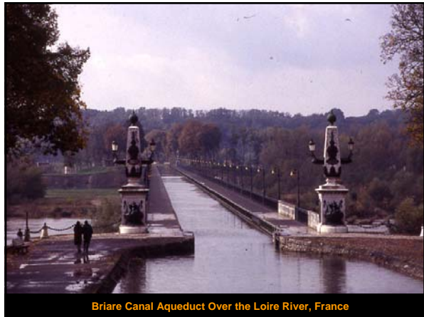
Briare Canal Aqueduct Over the Loire River, France
